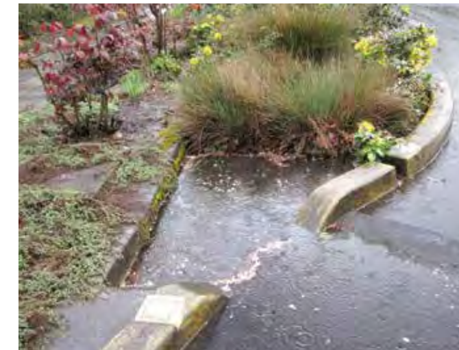
Bioretention facility in Spokane
